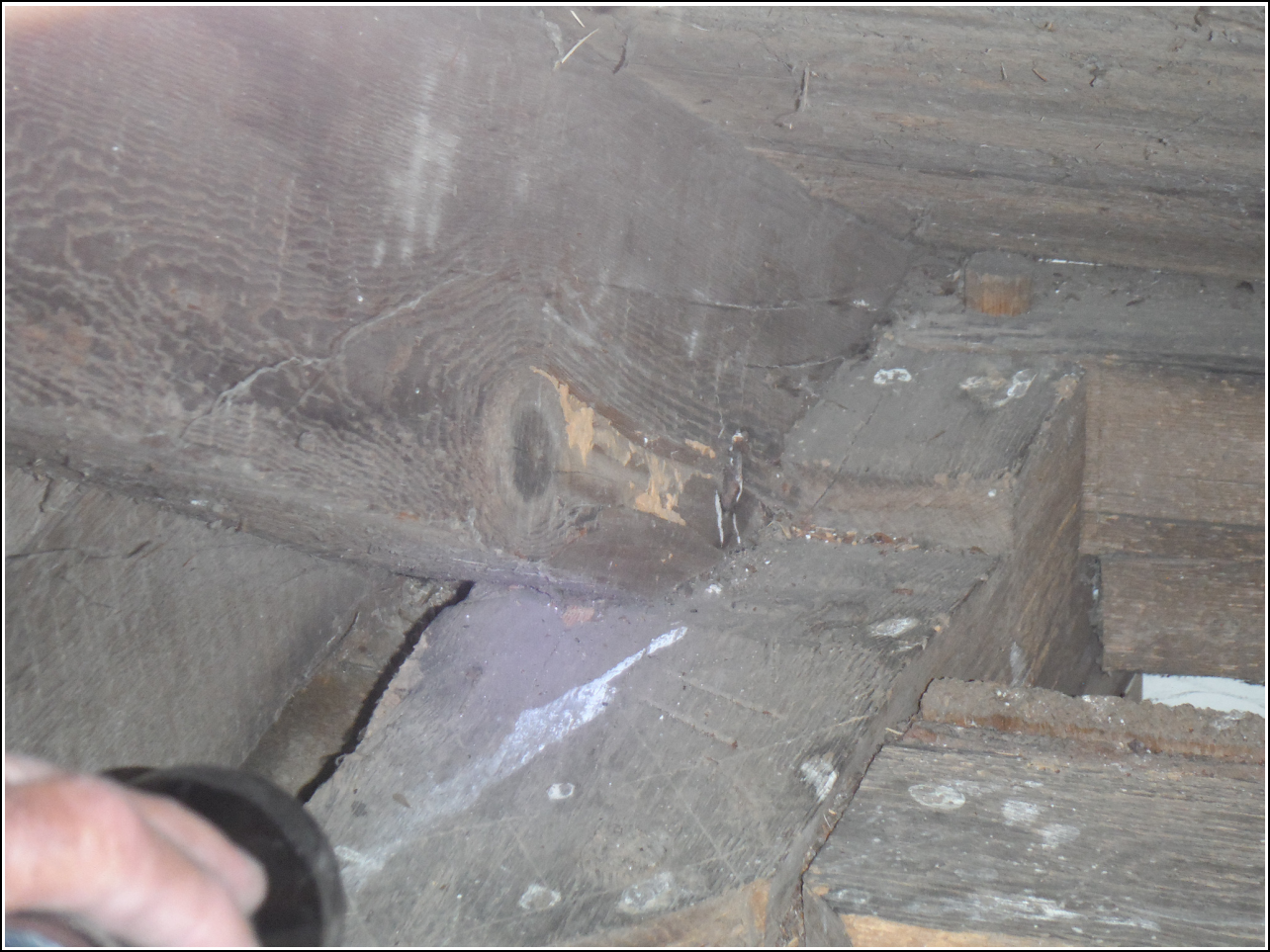
Figure 12. Carpenter drawing in attic at NW corner
