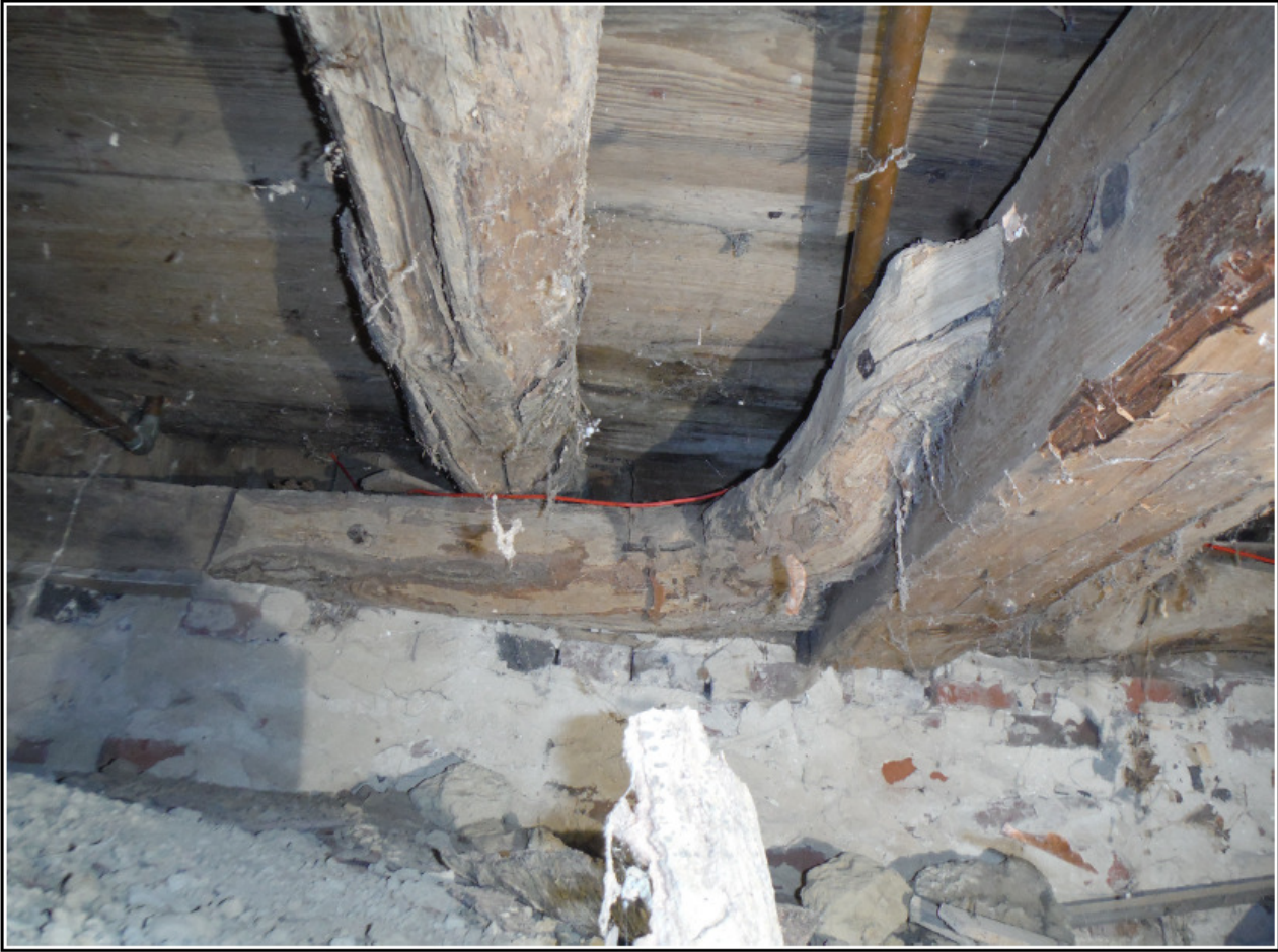
Figure 19. White oak ship's knee brace
