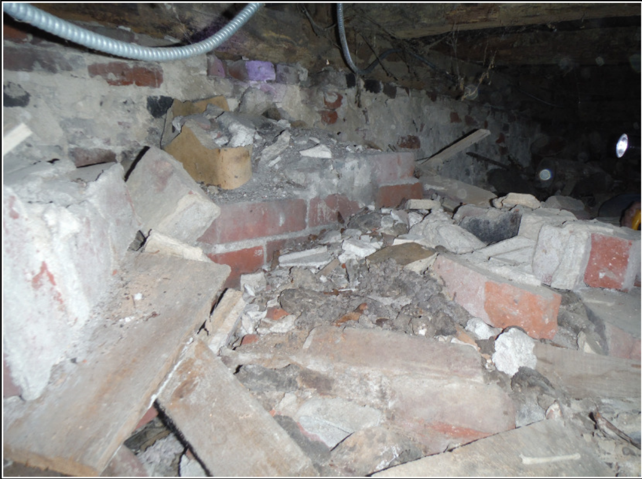
Figure 17. 20 th century chimney base in crawlspace
