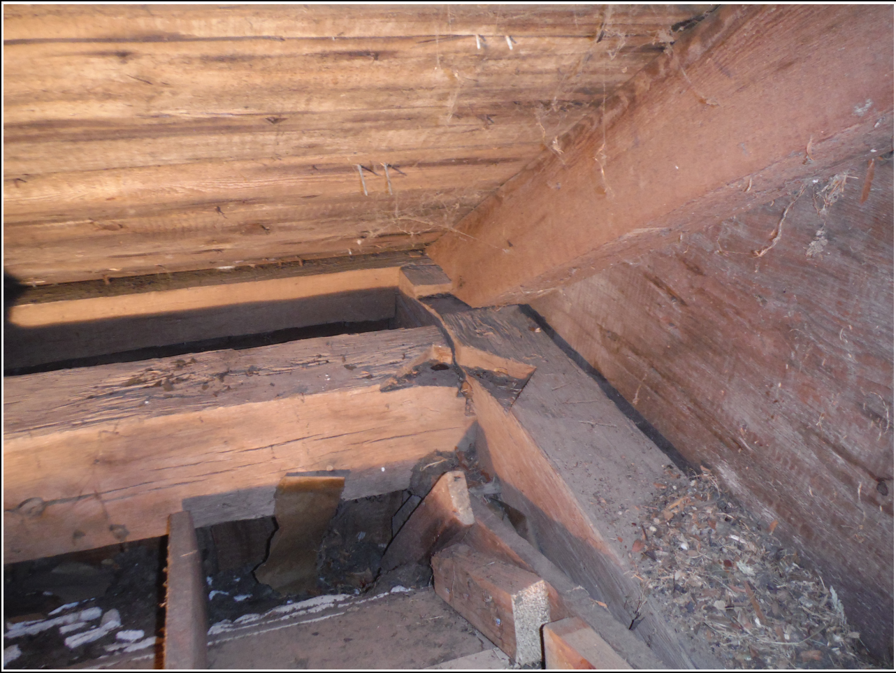
Figure 11. Pocket for original hip roof corner rafter
