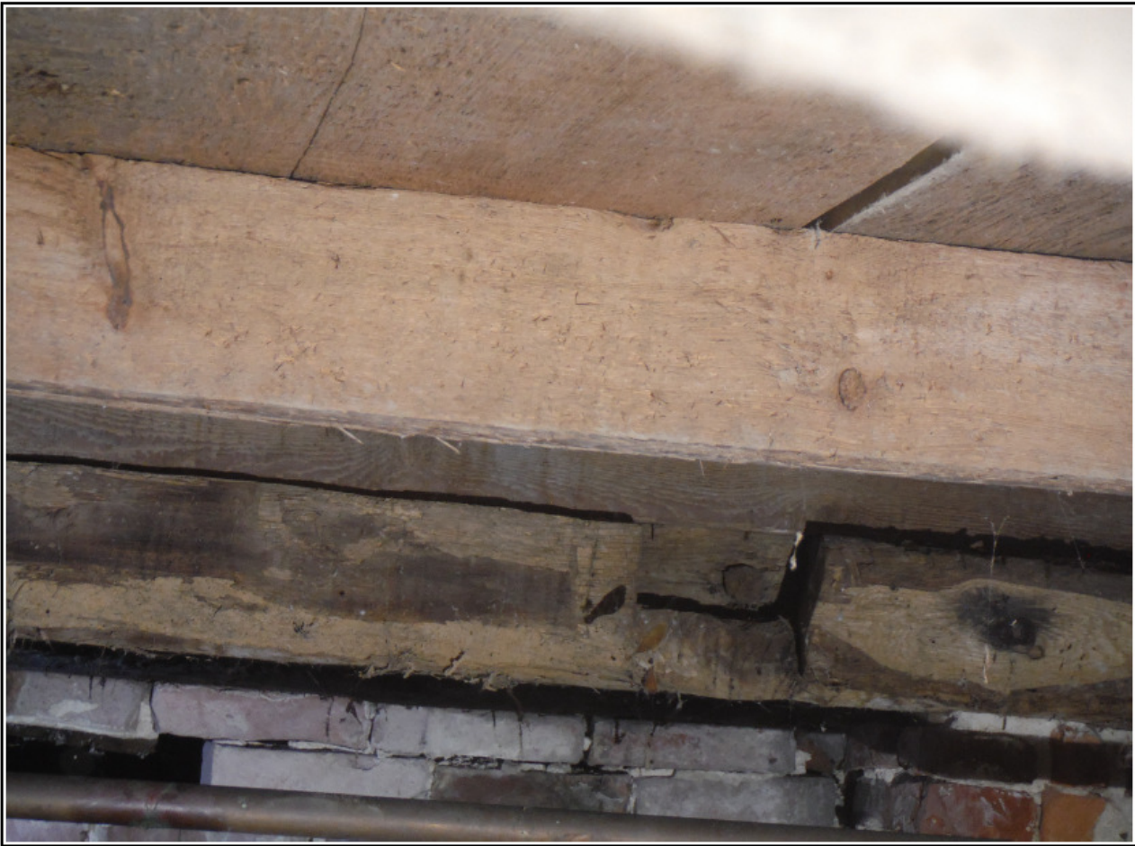
Figure 18. Original joist pocket in south sill
