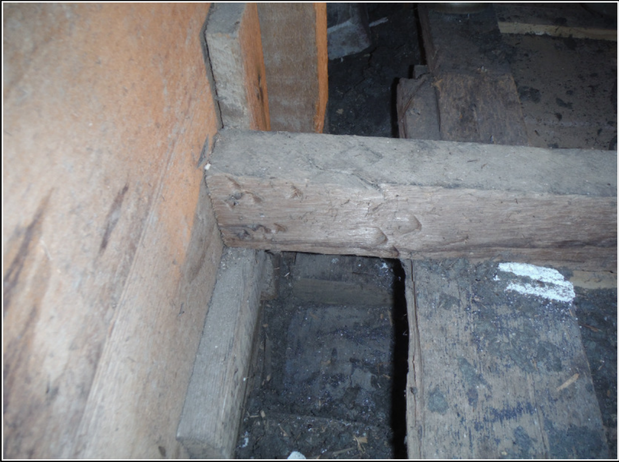
Figure 16. Girt mortise in attic
