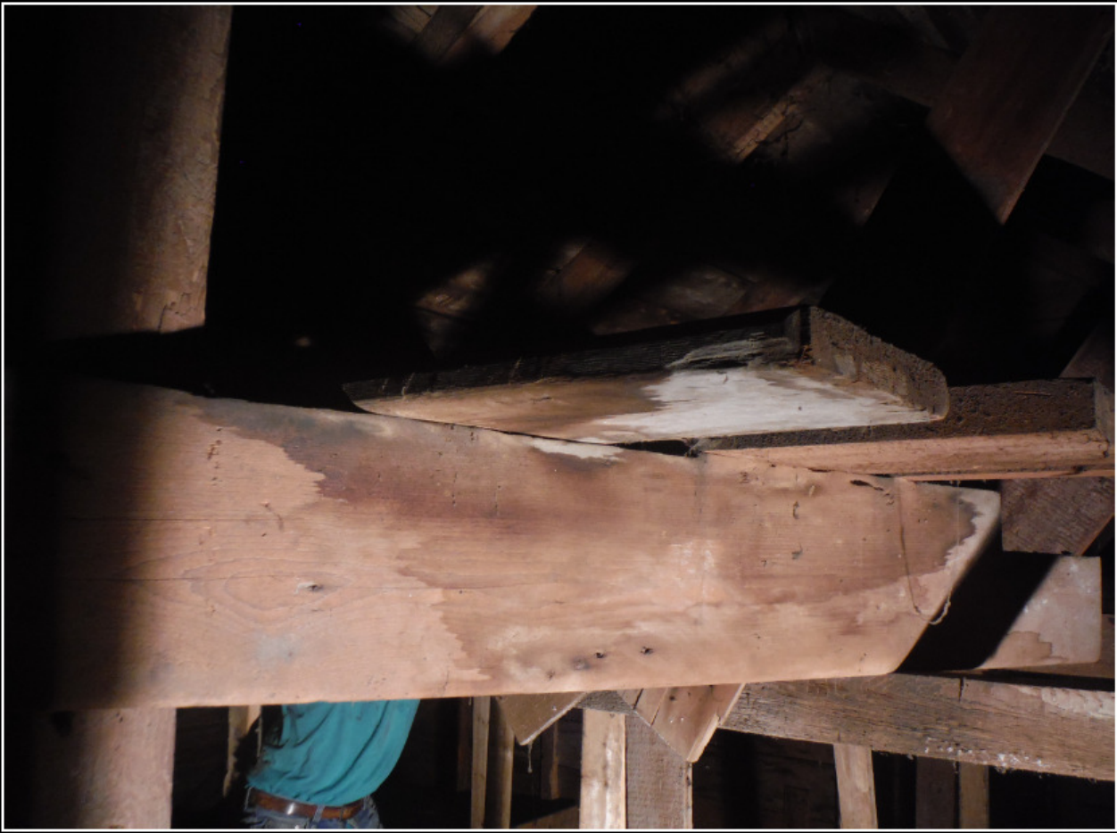
Figure 15. Platform made with reused risers beneath hole in roof
