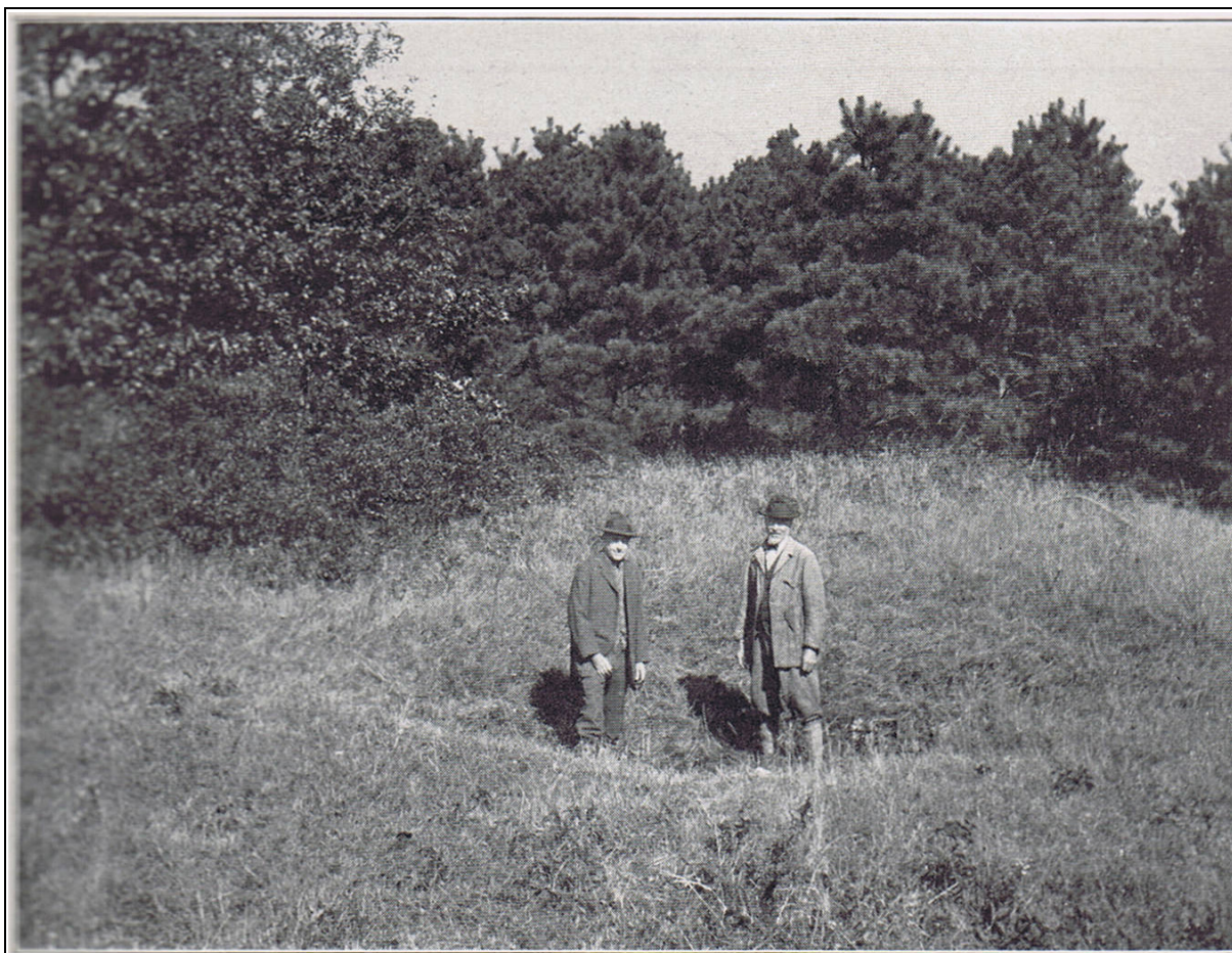
Figure 7. Lombard and Whitney at the start of the excavation
